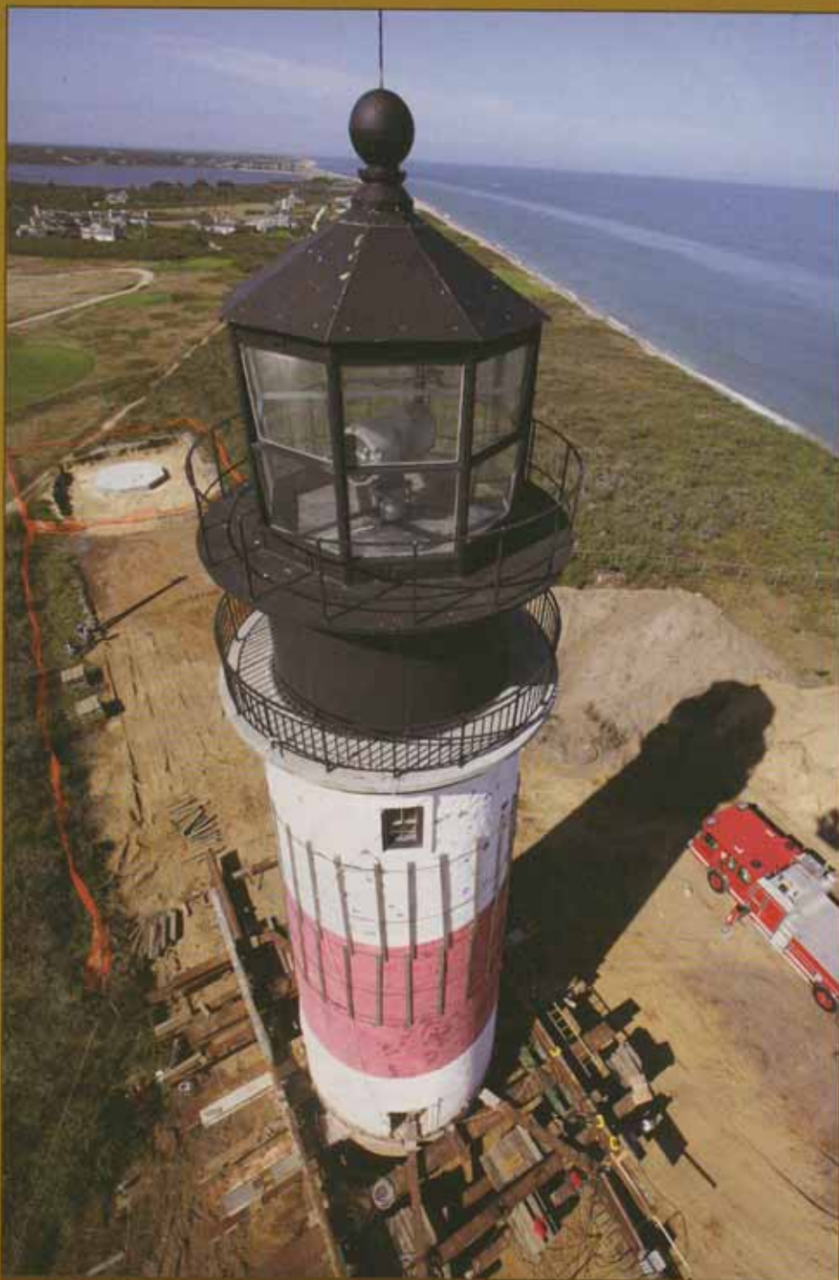
Sankaty Lighthouse "On the Move" as seen from atop the Nantucket Fire Department's Ladder Truck. Photo by Rob Benchley, courtesy of the Sconset Trust.
