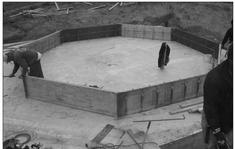
Spring work: the lighthouse is prepared and the new foundation is laid. Photos courtesy of Steve Scyok/International Chimney.
