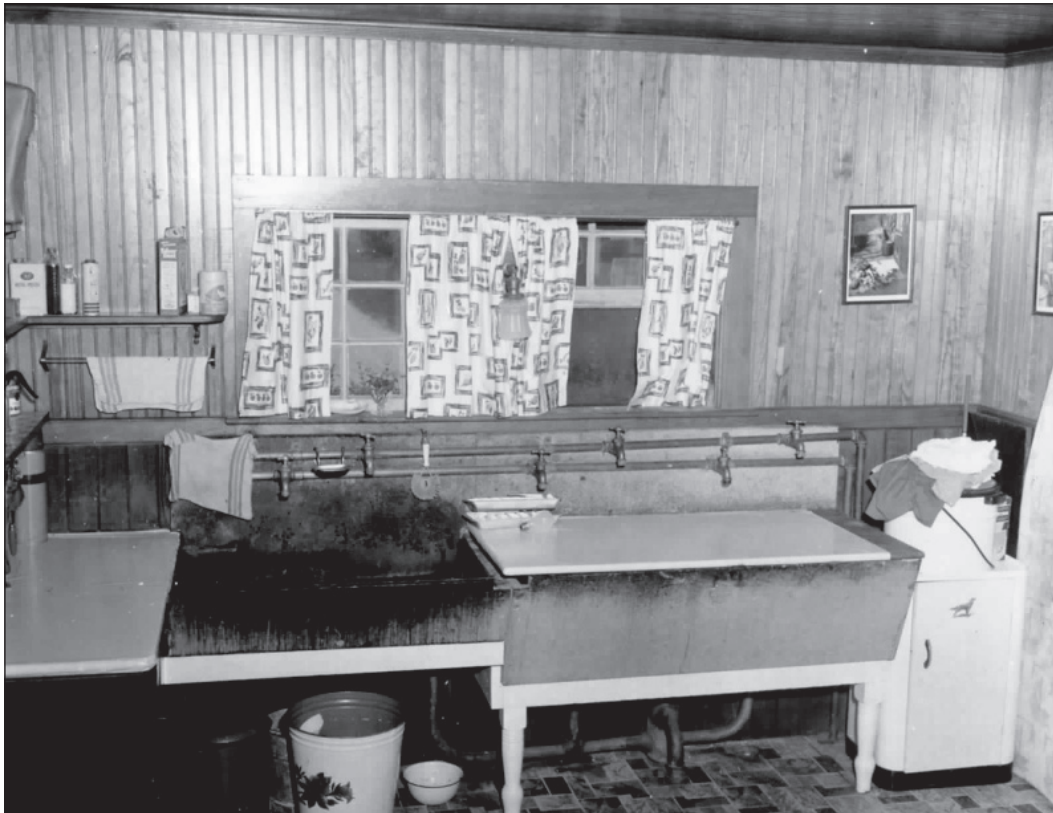
Kitchen original soapstone sinks
