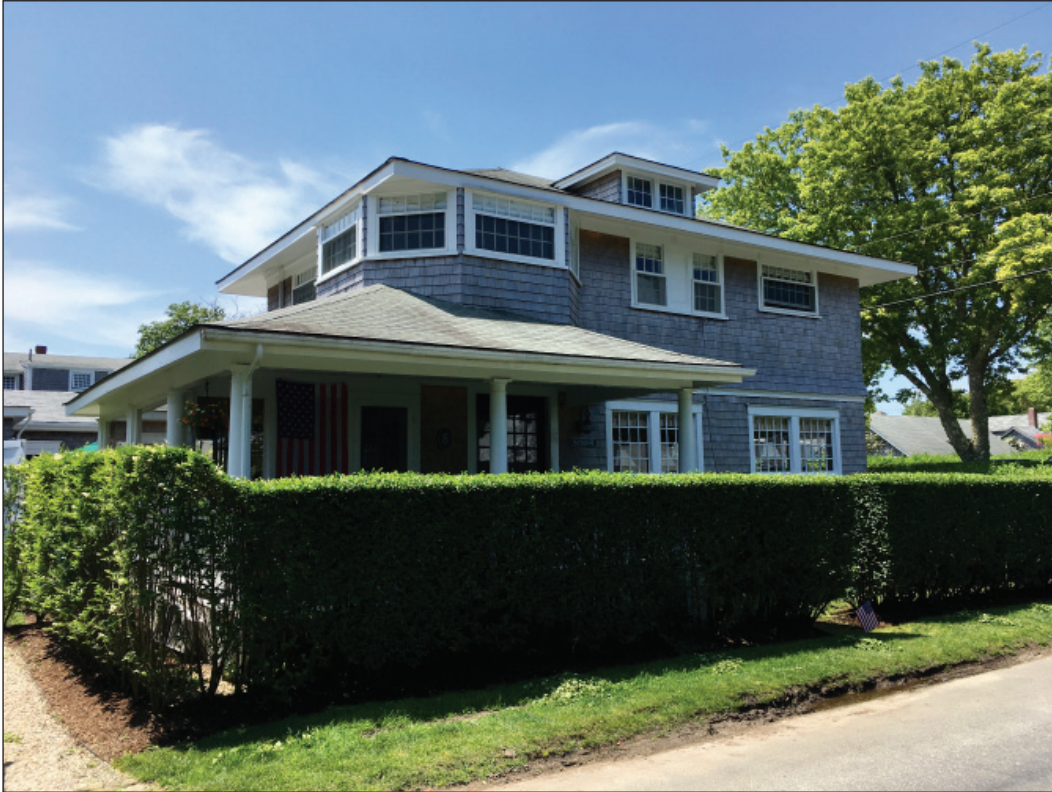
North & east streetfront elevations showing the wrap-around porch and the 'Pilot House'
