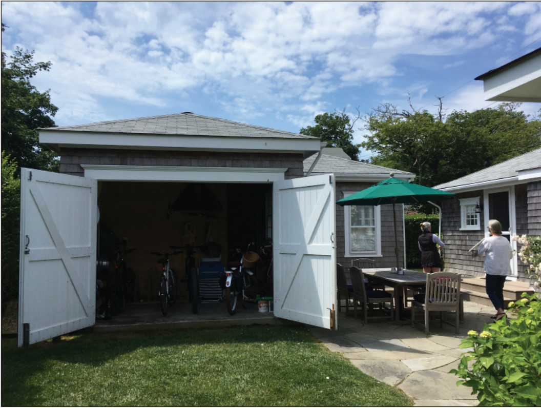
North elevation of Garage
