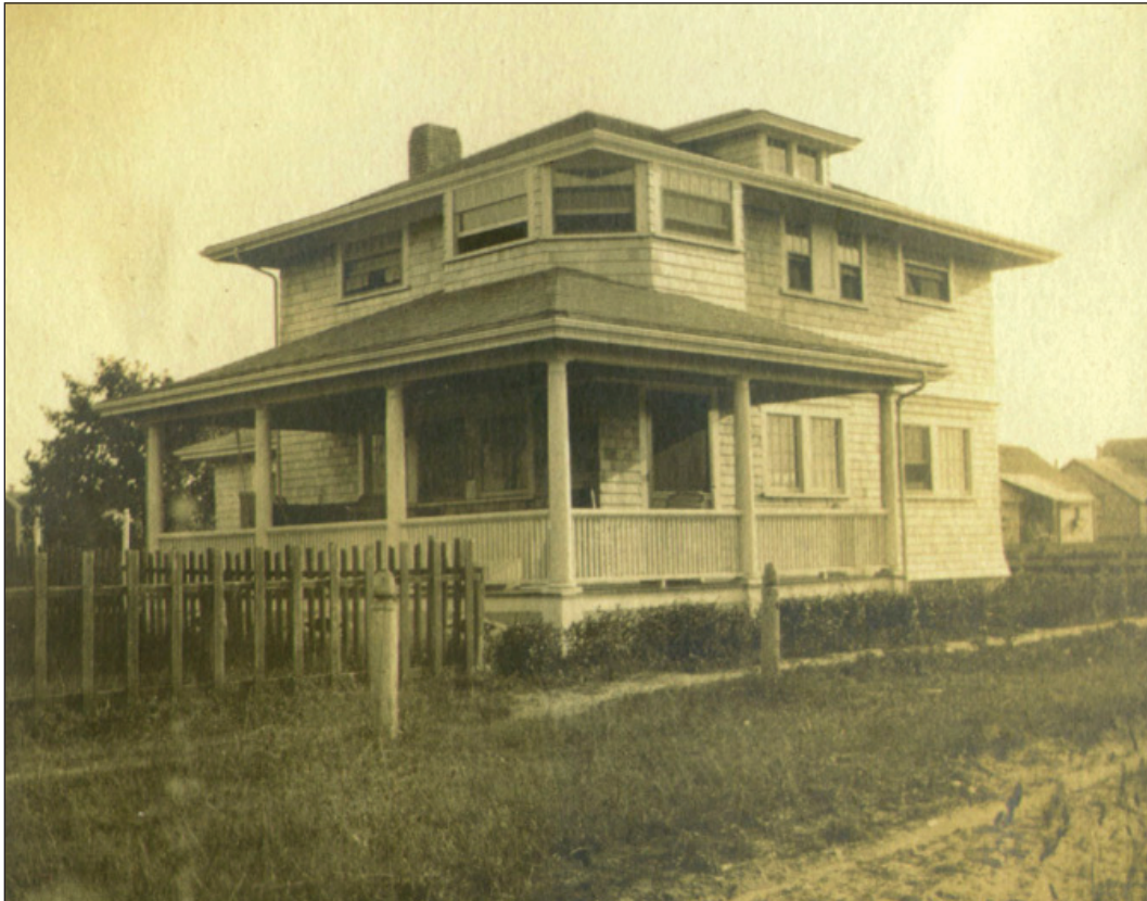
P20641: This photo shows the wrap-around porch at the northeast corner before the east portion was closed in.
