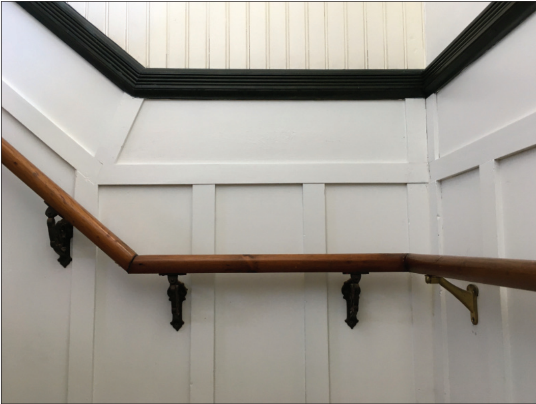
Stair wainscot, handrail & decorative handrail supports
