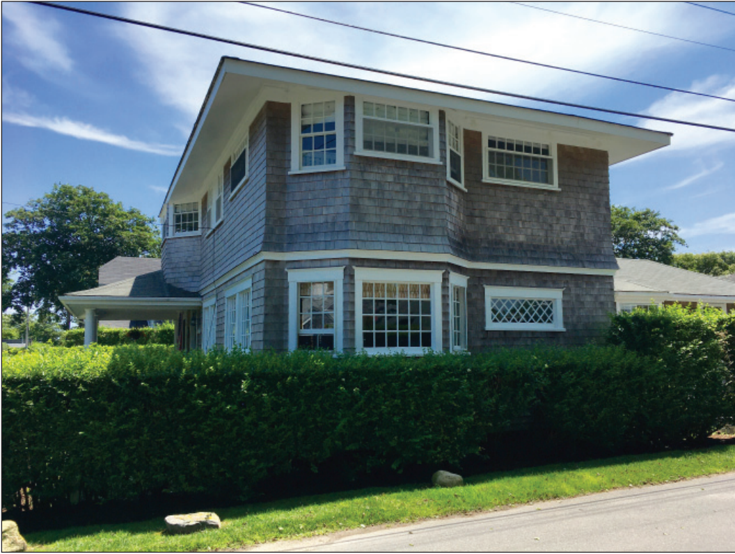
Partial west elevation showing 2-story bay window
