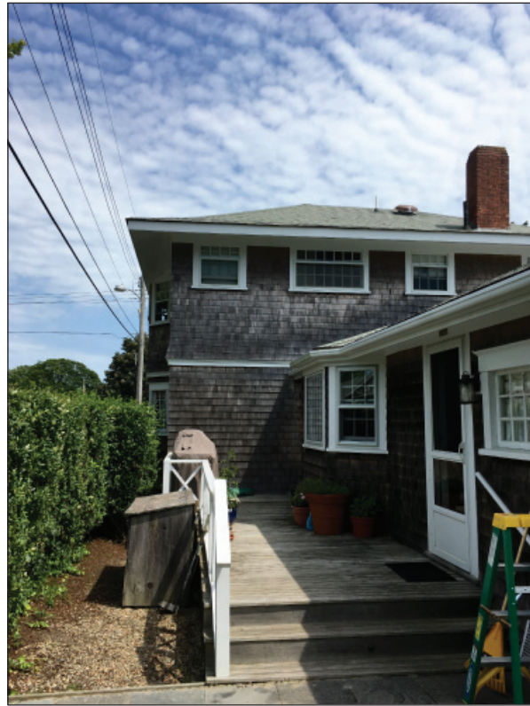
South elevation and west entrance deck
