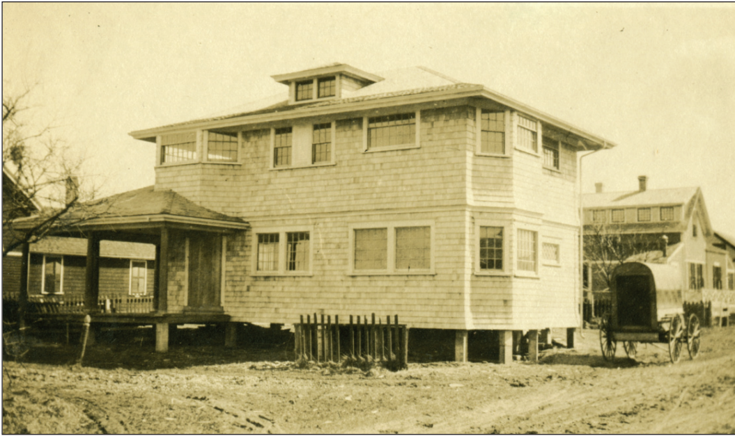
P10111: Ca. 1910, looking south at the north and west elevations. The house is shown with pier supports and square porch columns. The house may have been under construction at the time of this photo.
