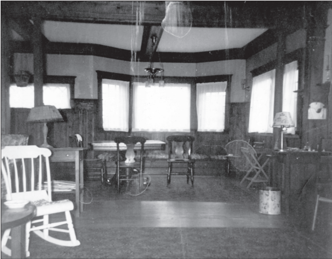
Dining Room Bay Window showing originally-unpainted wainscot woodwork
