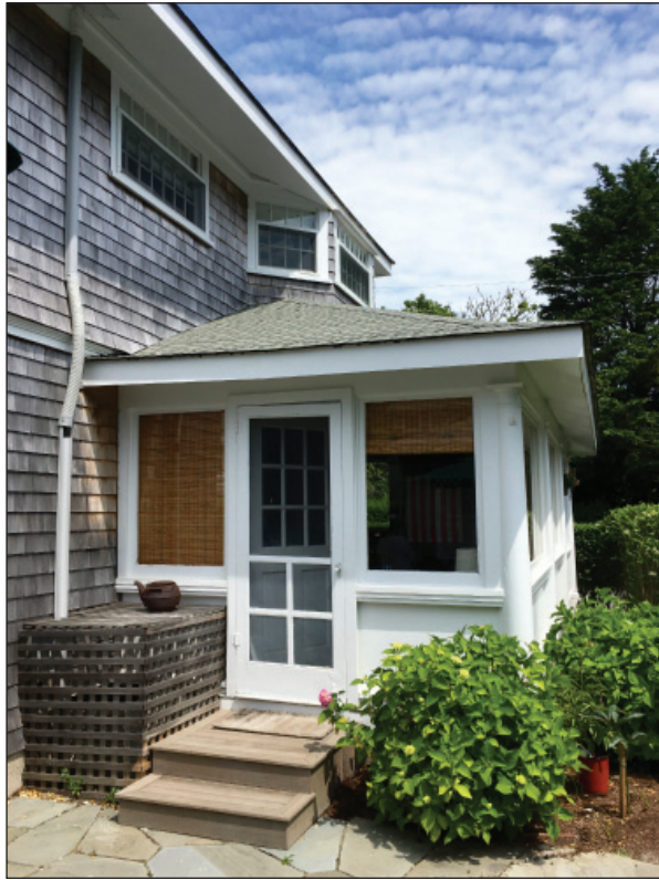
Partial west elevation showing enclosed east porch
