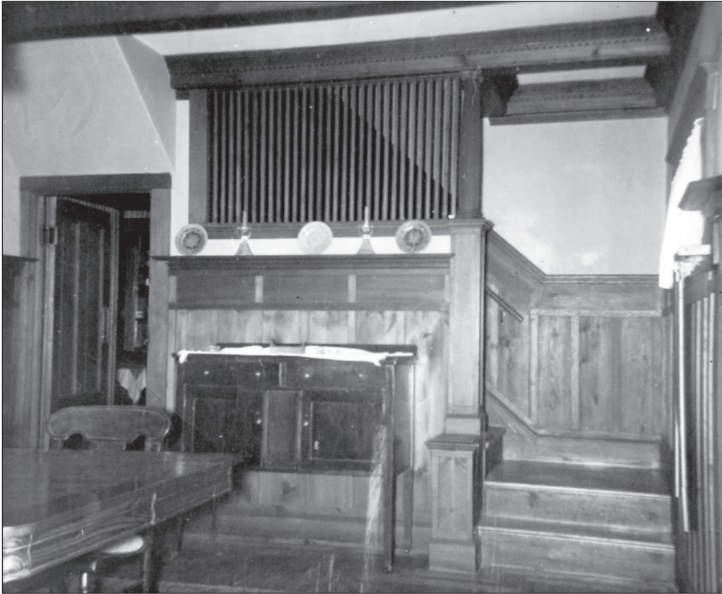
Staircase showing originally-unpainted wainscot woodwork
