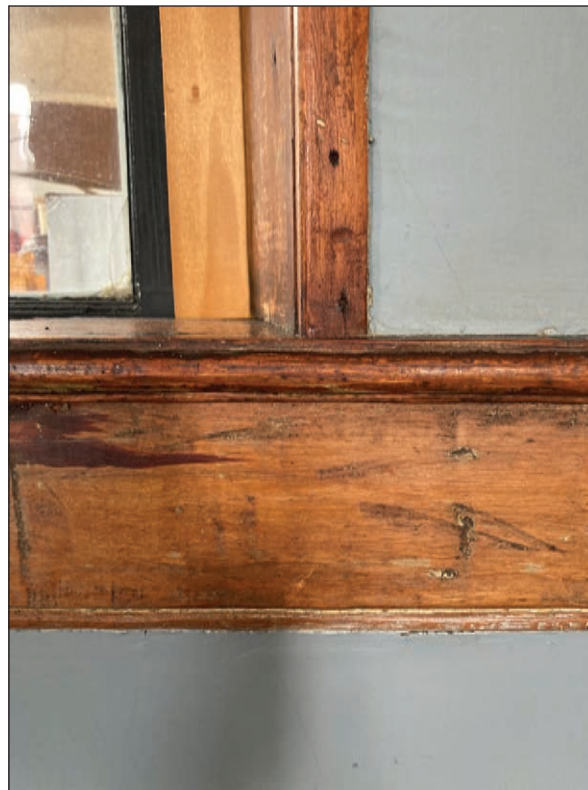
West Room Chair rail and Window Detail
