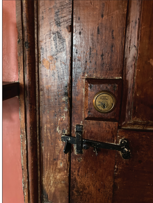
Door Trim and Thumbblatch Detail, East Room
