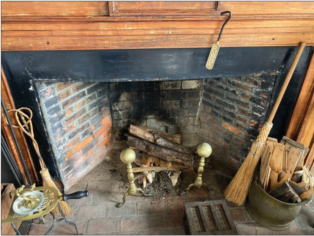
West Room Fireplace and Hearth
