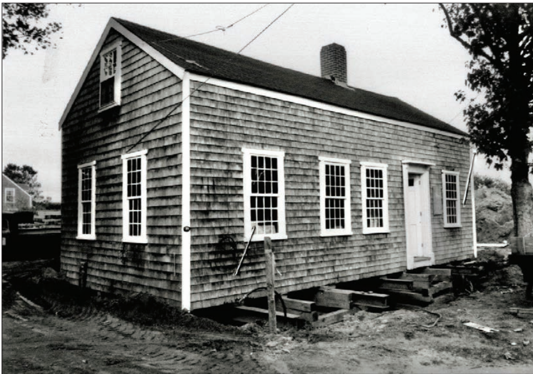
West and South Elevations during 1989 renovation
