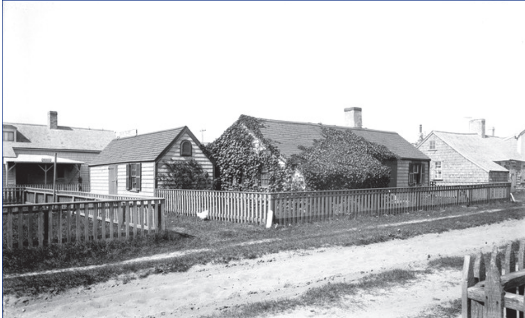
GPN2473: East elevation, 2 Center Street, left side, behind
