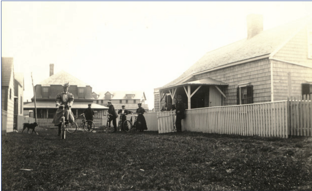
P3773: Looking south on Center Street, 1890s
