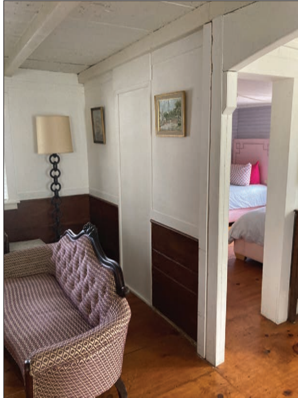
Original Plank Partition Wall with Closed-off Door
