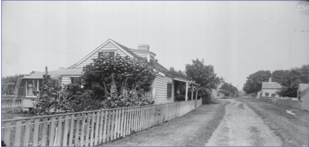
GPN3302: Looking north on Center Street, south and east elevations, late 19th-century additions, painted white
