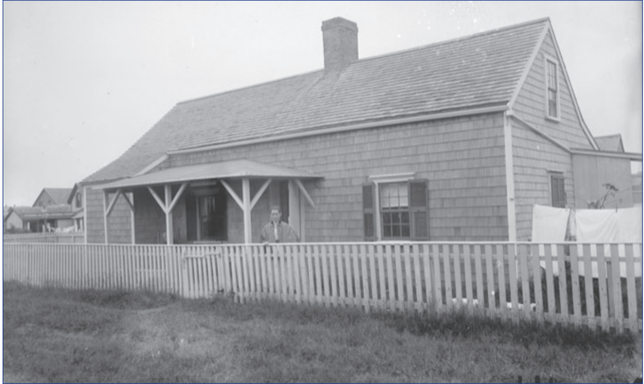
GPN3301: East Elevation showing the porch addition
