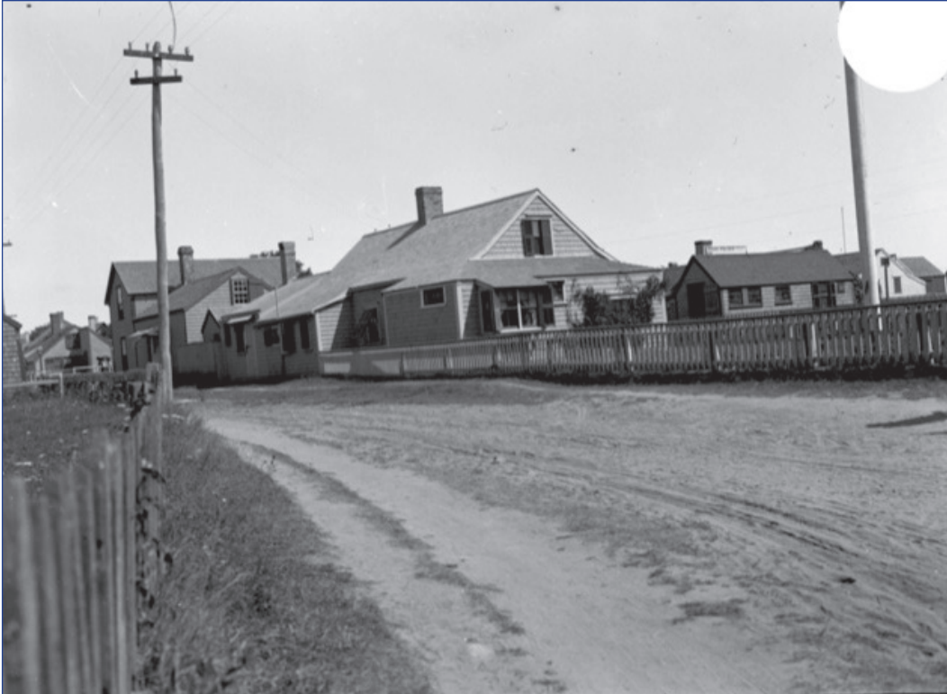
GPN3201: Looking northeast on Shell Street, 1920s. Note telephone poles
