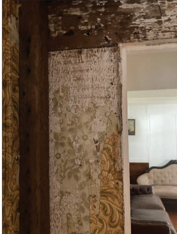
Dining Room, Wallpaper Remnants
