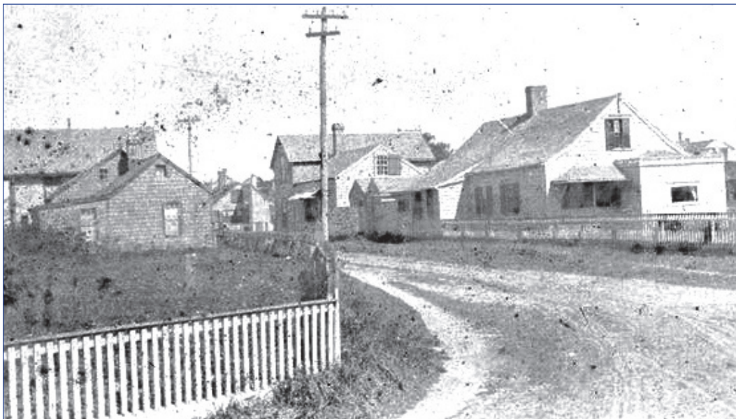
PH53-36: Looking north on Shell Street, west and south elevations, showing early south additions
