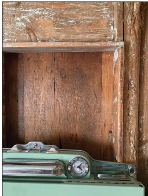
Kitchen earlier north window trim opening
