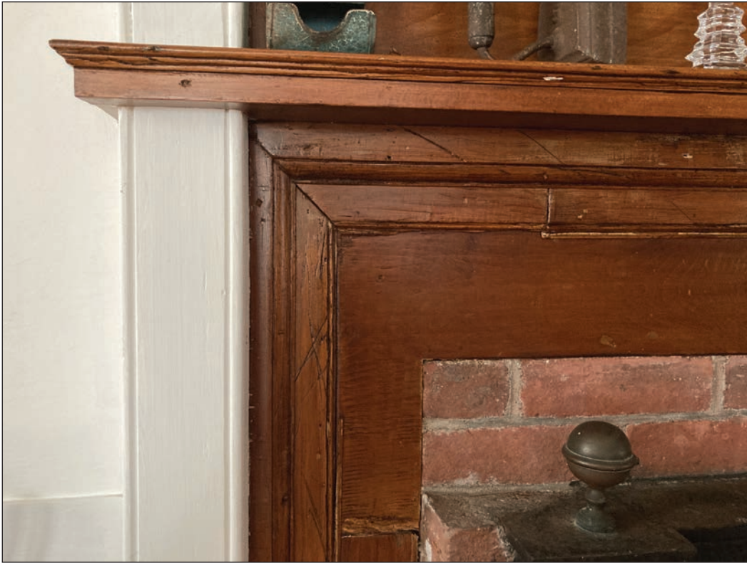
Chimney Mantelshelf and Moulding Detail
