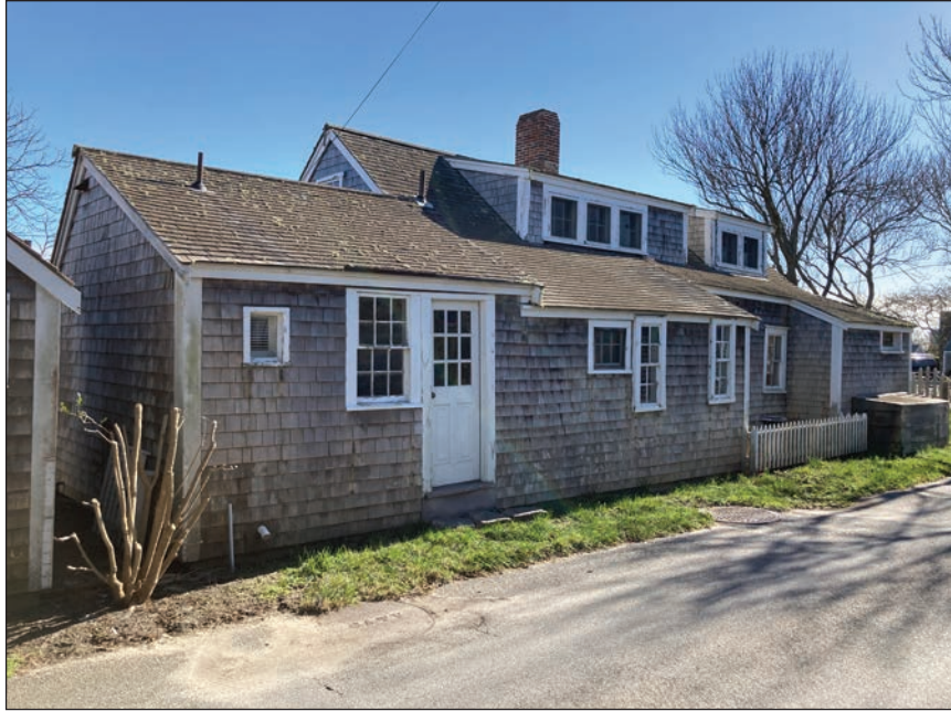
North and West Elevations
