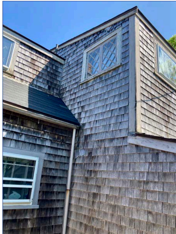
West side of Southeast second floor addition
