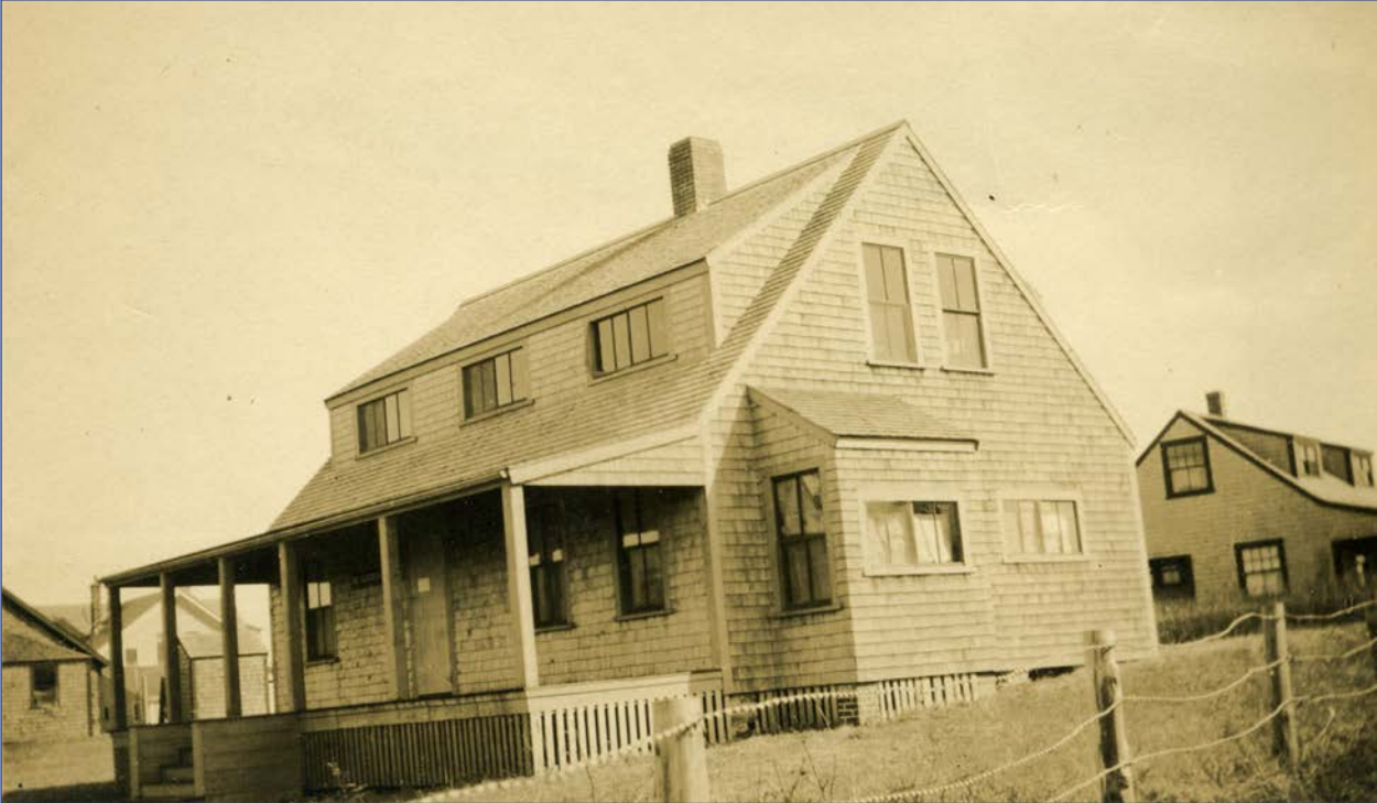
P10110: 10 Everett and 28 Morey, c 1910 North and West Elevations
