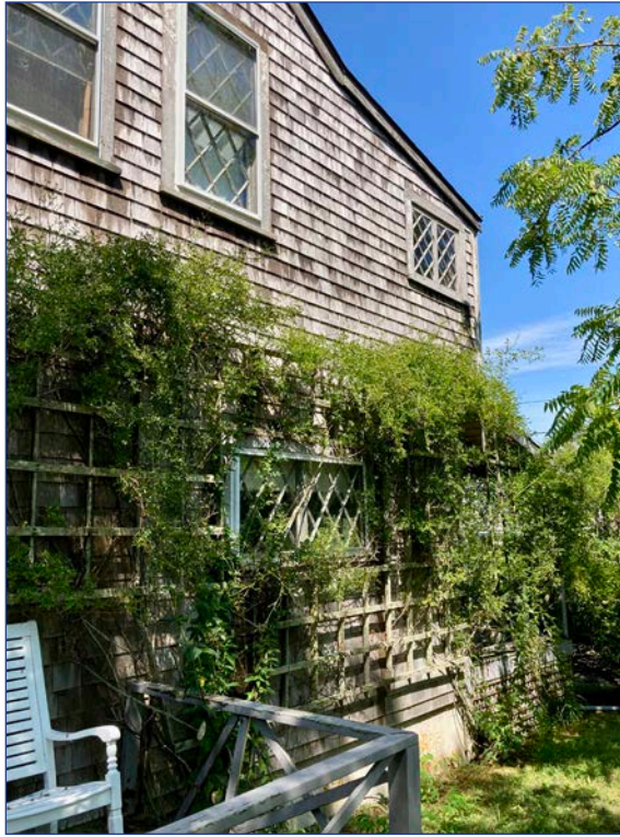
East Elevation looking North
