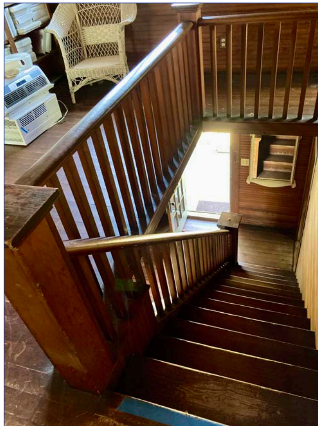
Stair to First Floor
