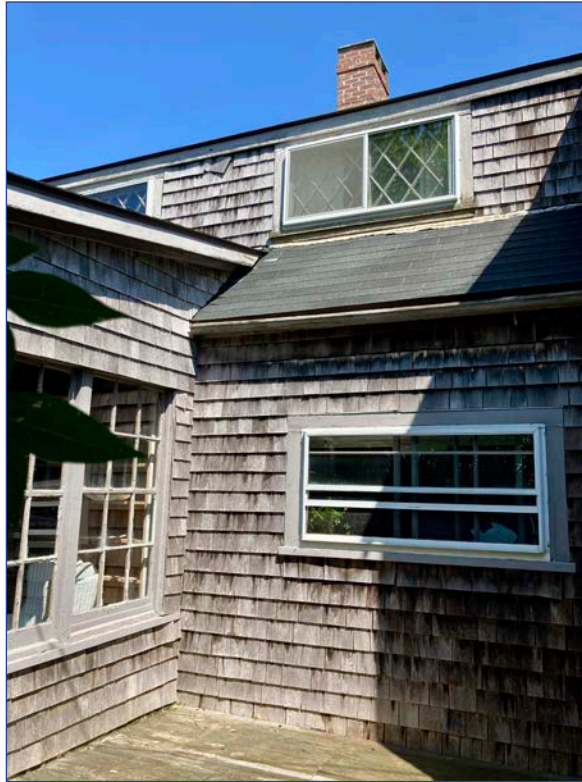
South & East Walls at South Deck
