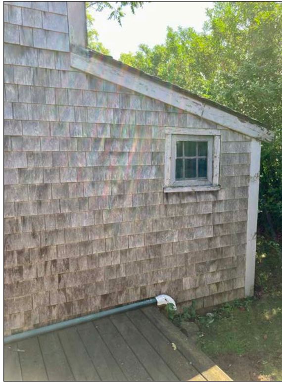
West side of Southeast corner Laundry Room
