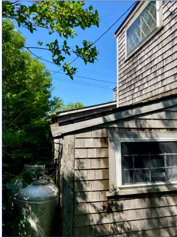
South side of East Elevation showing second floor addition
