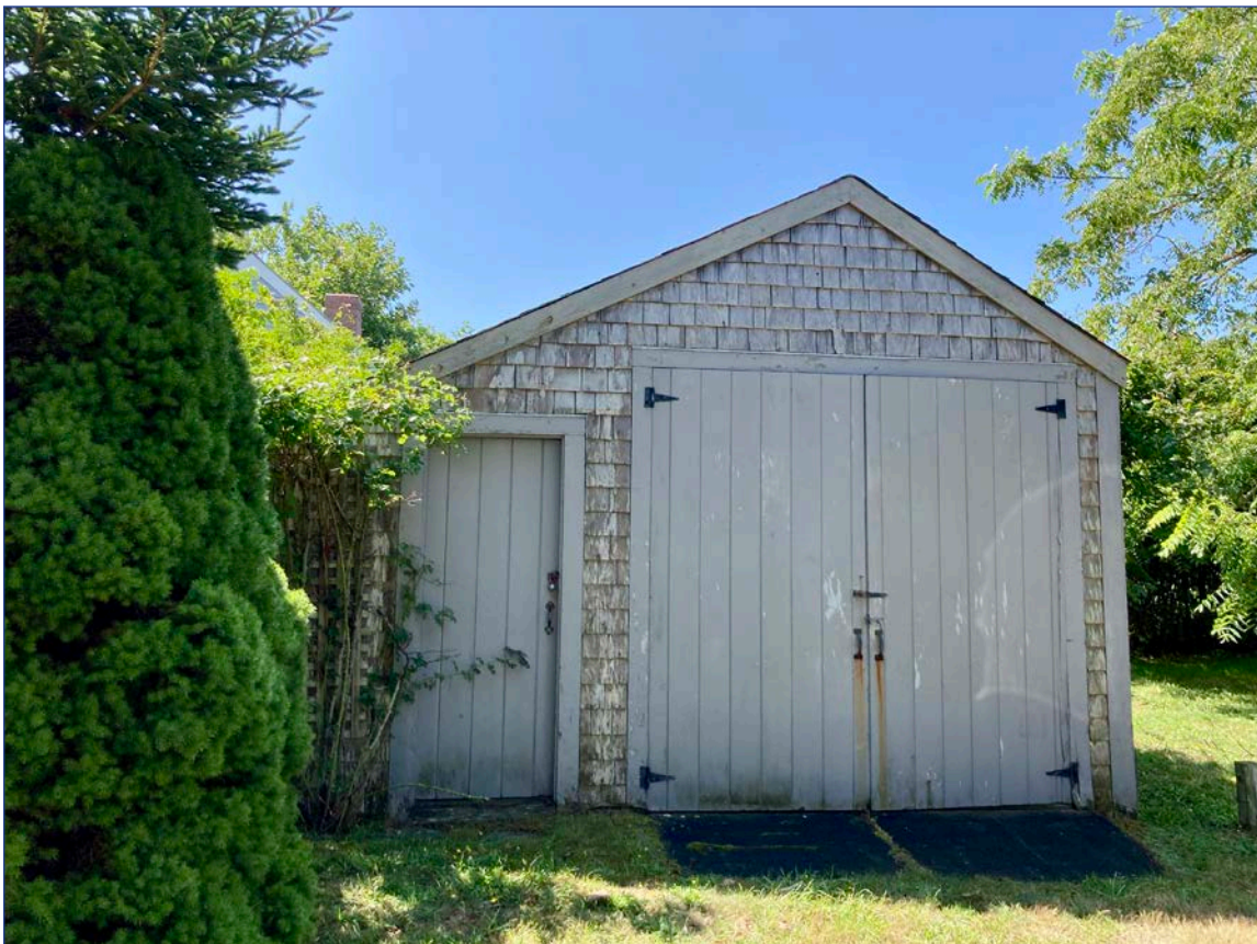
Garage, east end of house
