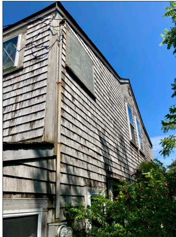
East Elevation Second Floor looking North
