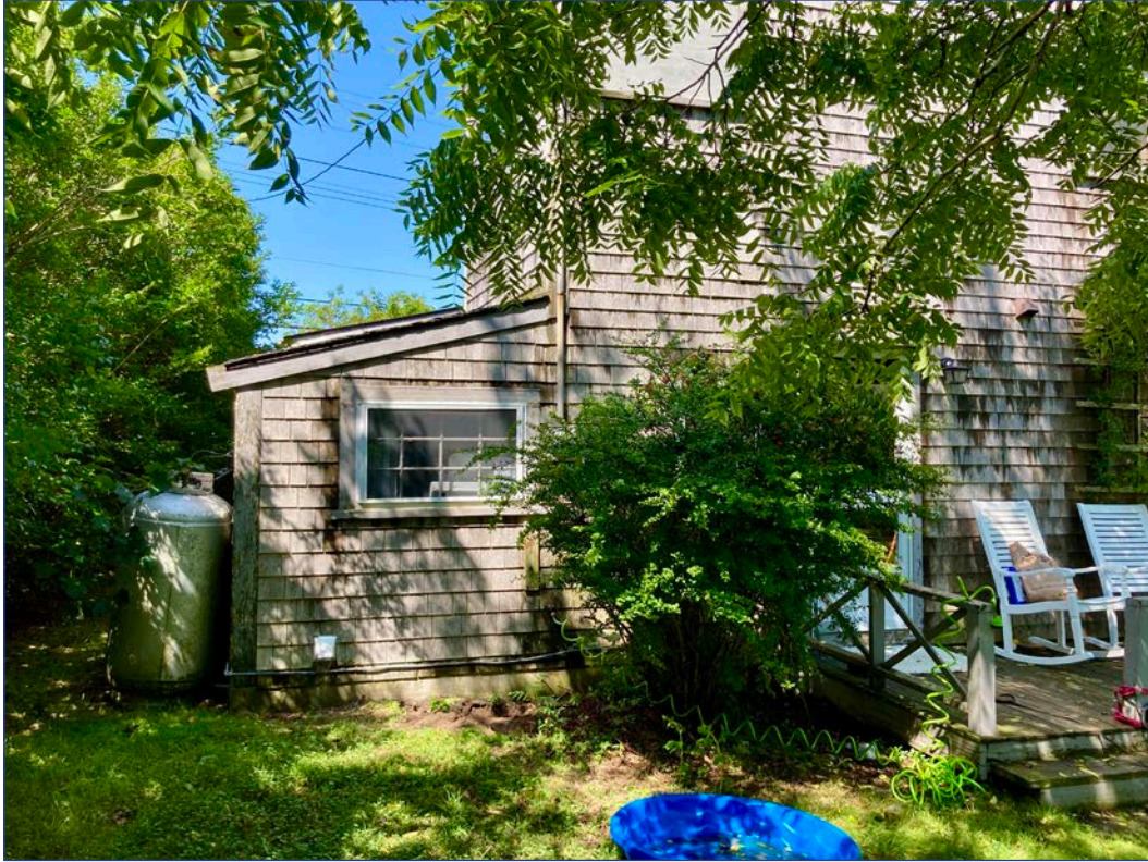
South side of East Elevation
