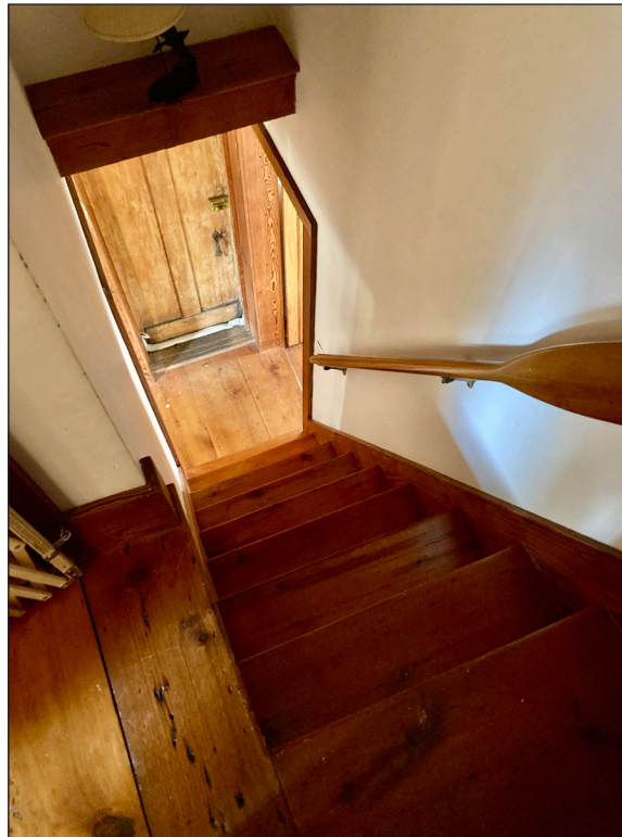
View Down the Stair
