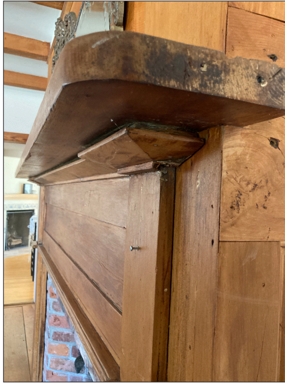
Moulding Detail: Fireplace East Front Room
