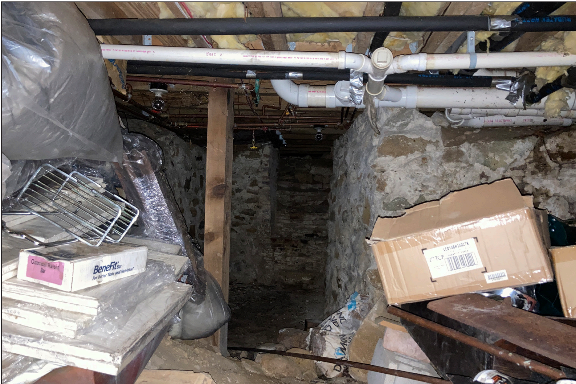
Basement View to Early Stone Foundation
