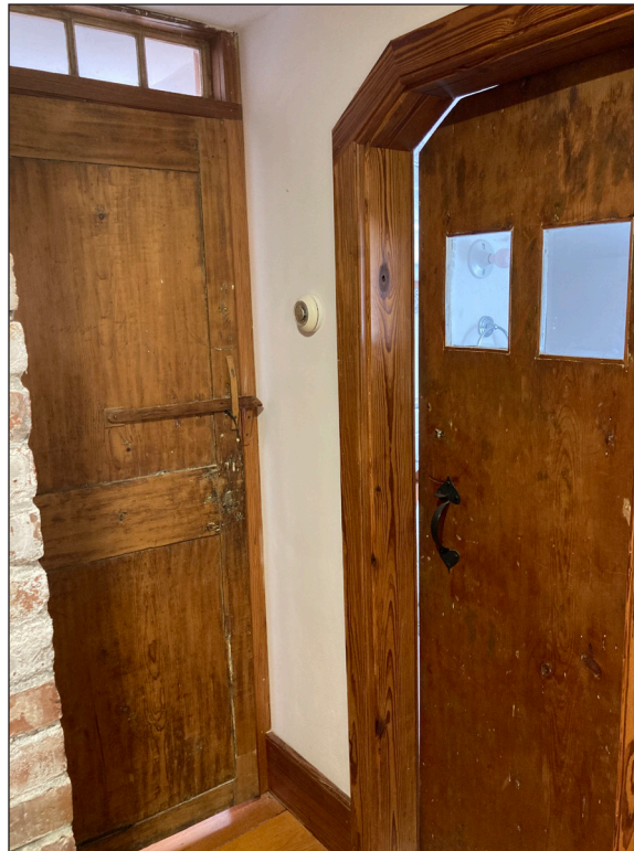
Stair Landing Second Floor
