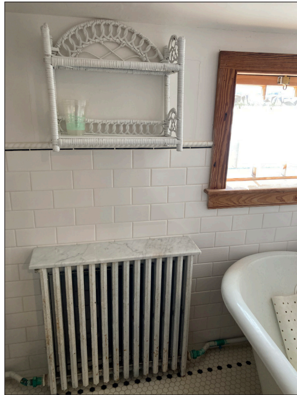
Second Floor Bathroom
