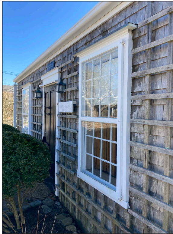
Front 12/12 Plank-Framed Window Sash
