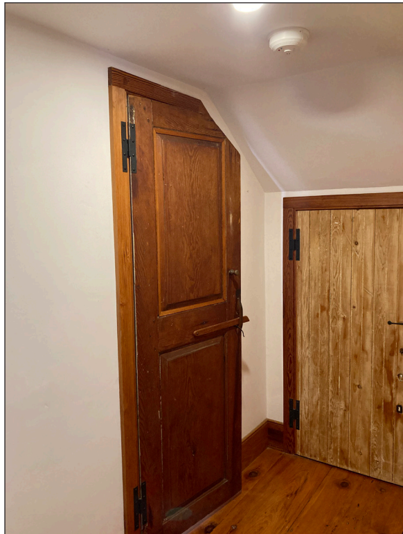
Stair Landing Second Floor
