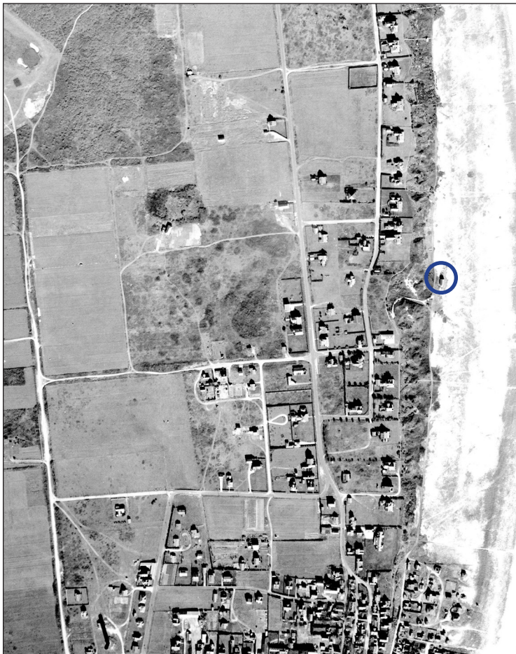
1935 Aerial, p8000, showing location of Massachusetts Humane Society building.
