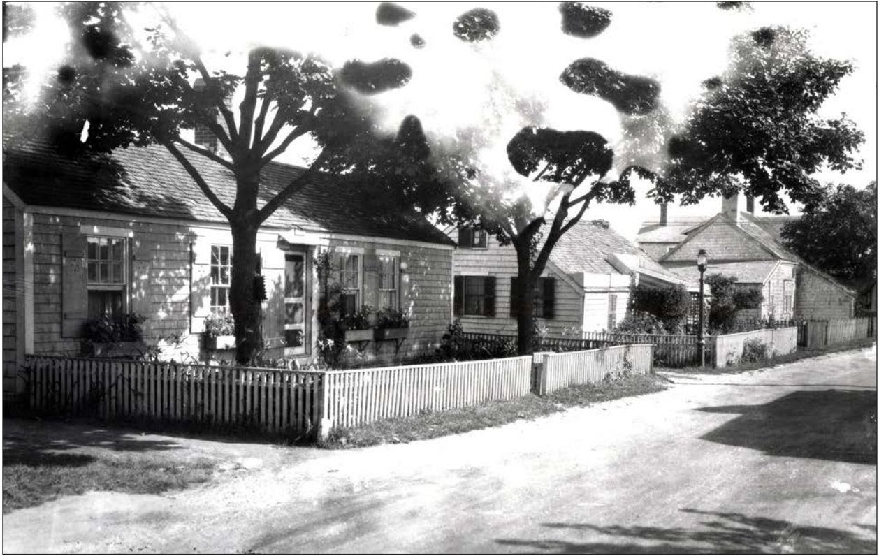
F770, 1920's, Looking south on Broadway (the third house), showing darker trim, a house to the north, possibly a paraged chimney
