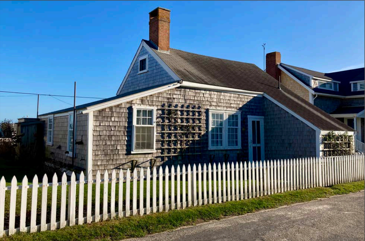
Broadway West and North Elevation
