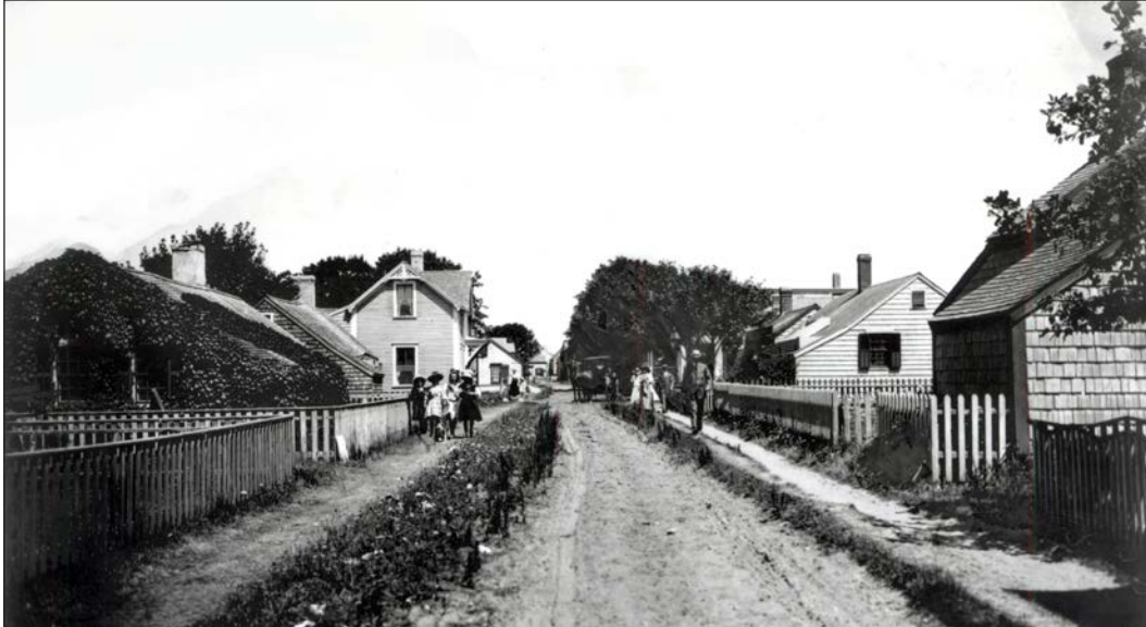
GPN4303, Looking northeast, first house on the right
