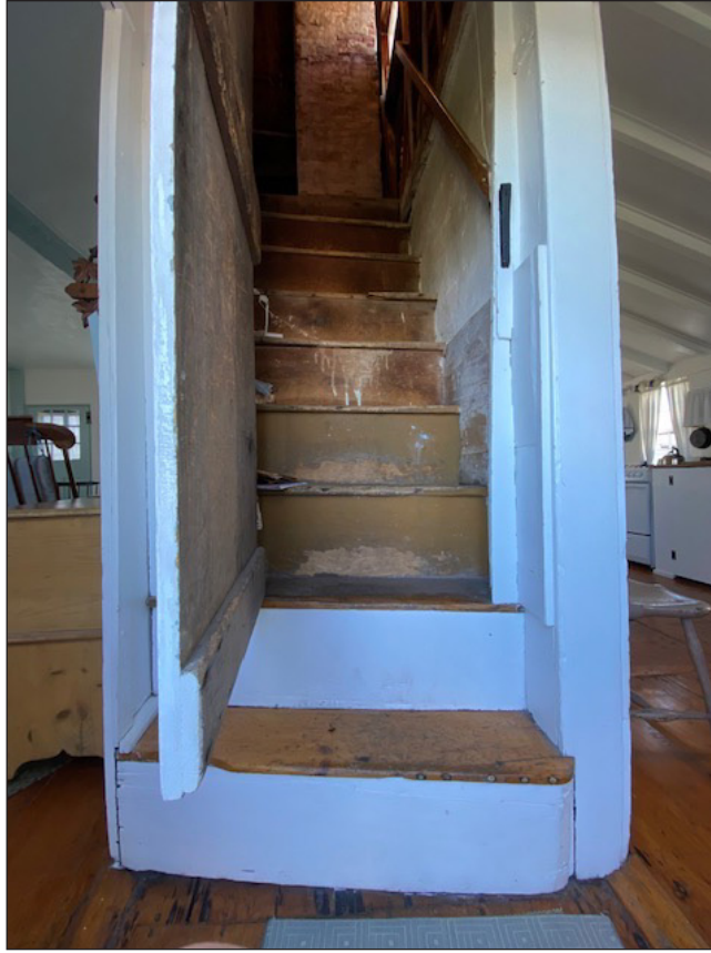
Stair to Attic
