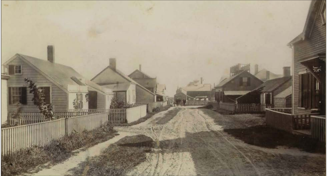
P2632, Looking south on Broadway (the second house on the left), showing a darker trim, a house to the north, possibly a parged chimney.
