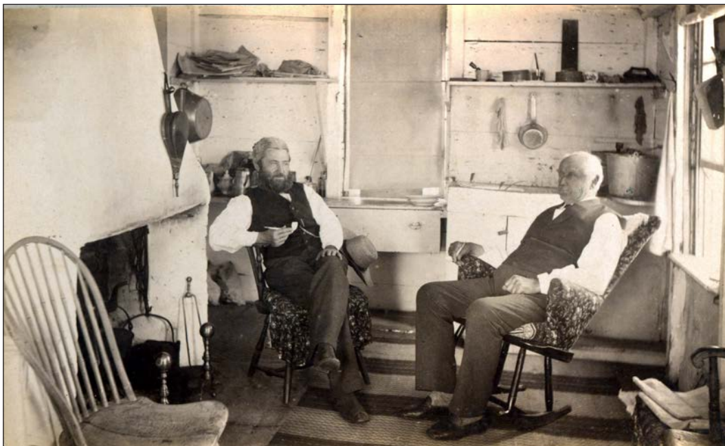
A15-24 (GPN3434), 1882, from "Old 'Sconset and along Shore" H.S. Wyer The wood kitchen drawer and sink cabinet shown in this photo have survived. Changes include a larger sink, a refrigerator in the corner, and the removal of the fireplace masonry. What now remains are the angled brick sides.
