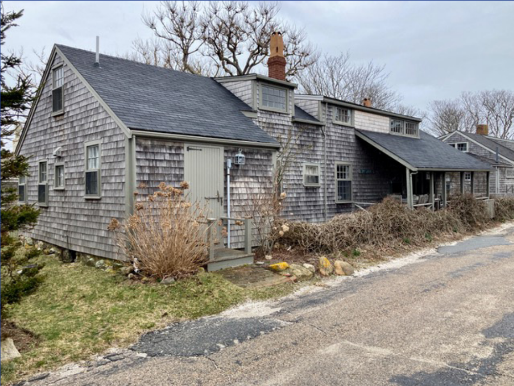
South and East Elevations
