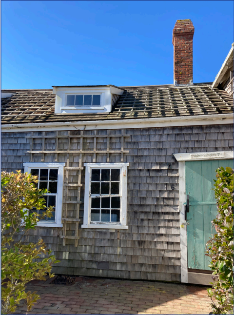
Center Street East Elevation
