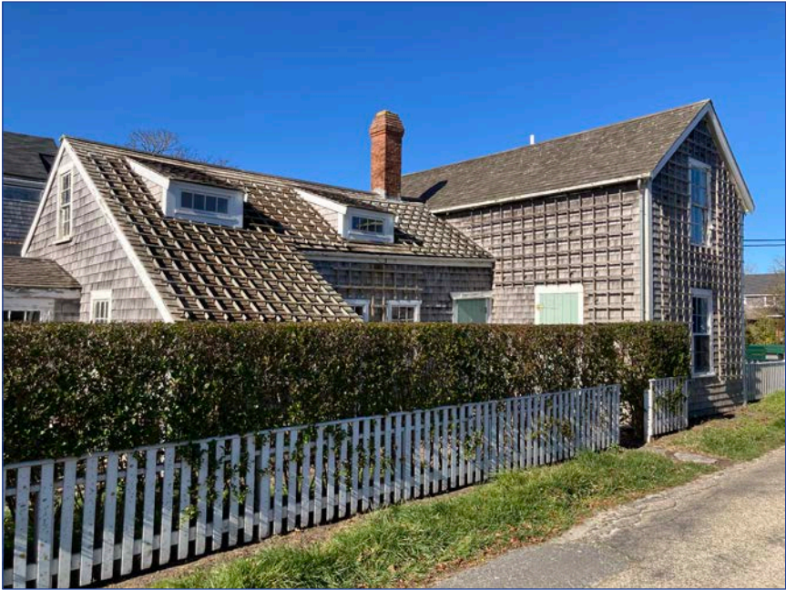
Center Street South and East Elevations
