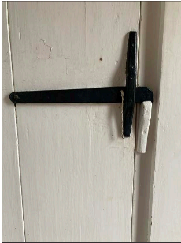
Board-and-Batten Door with Lift Bar Assembly
