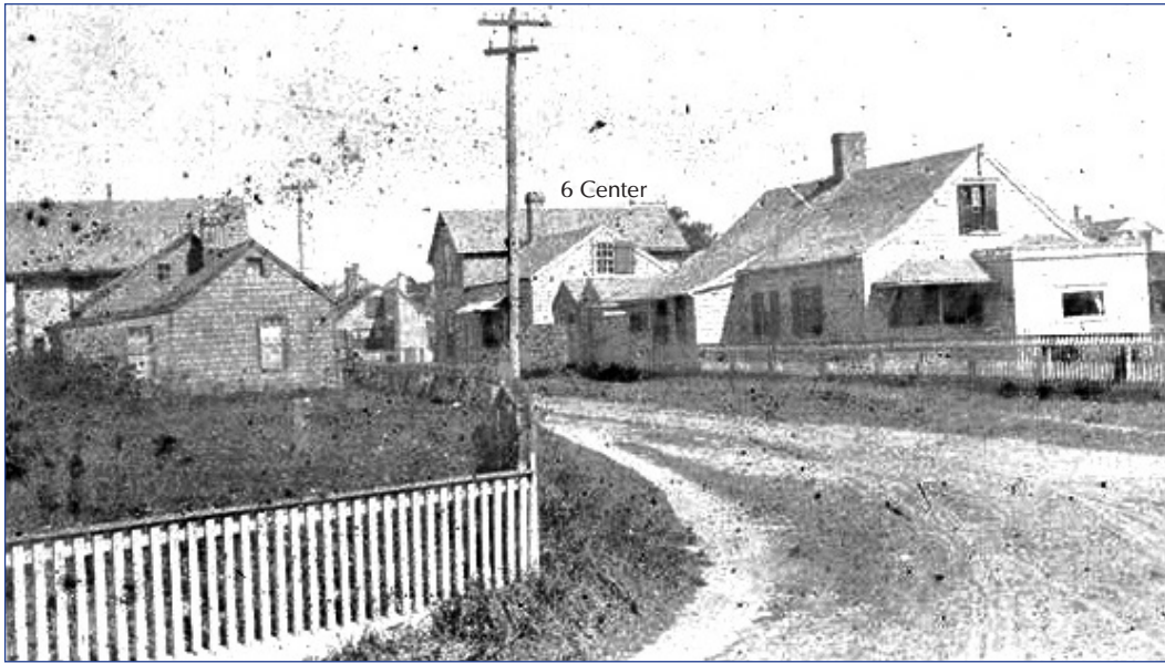
PH53-36: Looking north on Shell Street, west and south elevations, showing early south additions
