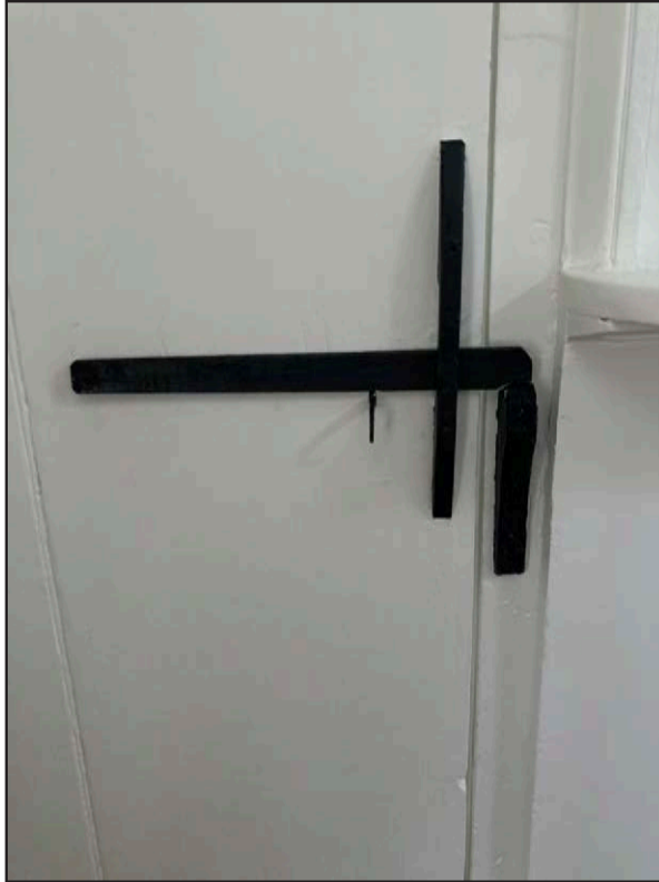
Board-and-Batten Door with Lift Bar Assembly
