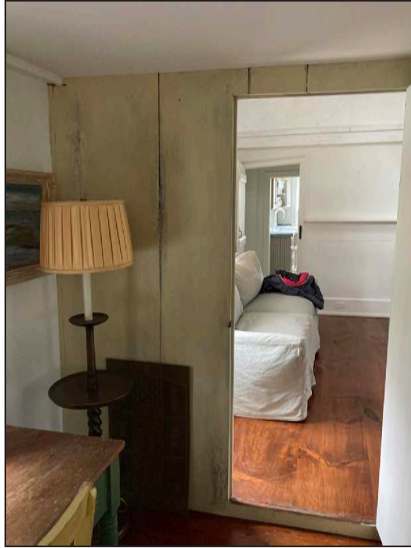
Vertical Plank Interior Wall Between Living Room and Bedroom
