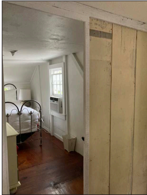
Vertical Plank Interior Wall in Bedroom
