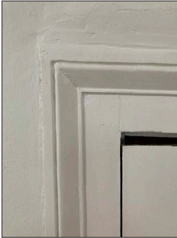
Early/original Door Trim Moulding in Living Room
