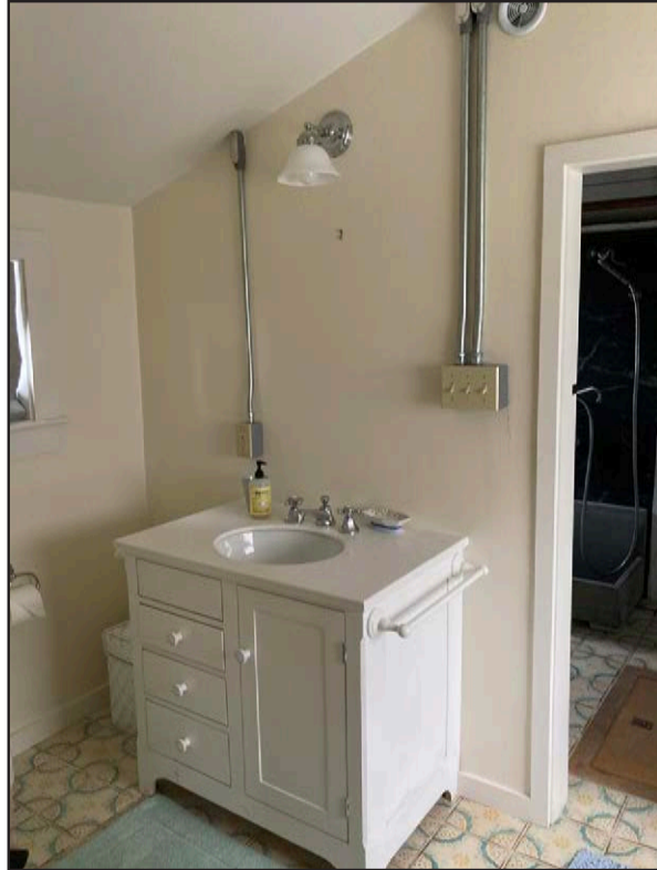
First Floor Bathroom
