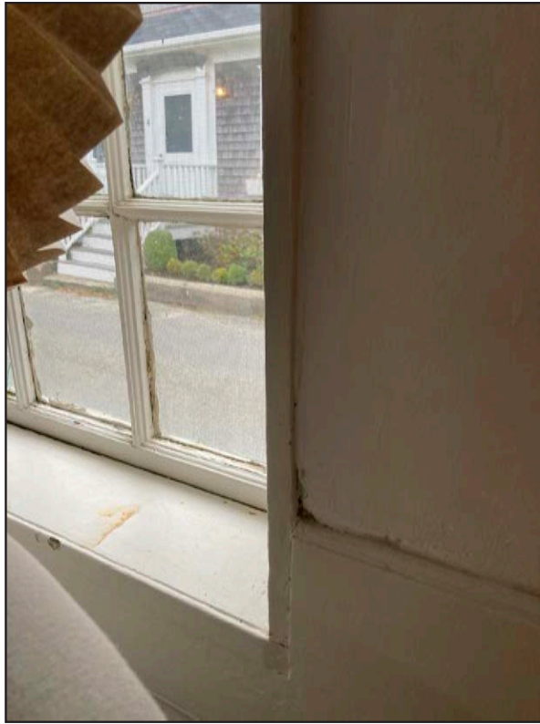
Early Typical Window Casing
