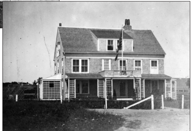
SC612-25, Penrose Cottage, 3 Grand Avenue, 1920s
