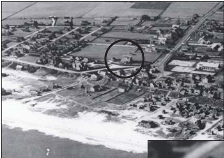
NHA_F4097 1926 Aerial Photo The Ocean View House as a 20th-century residence including a garage.
