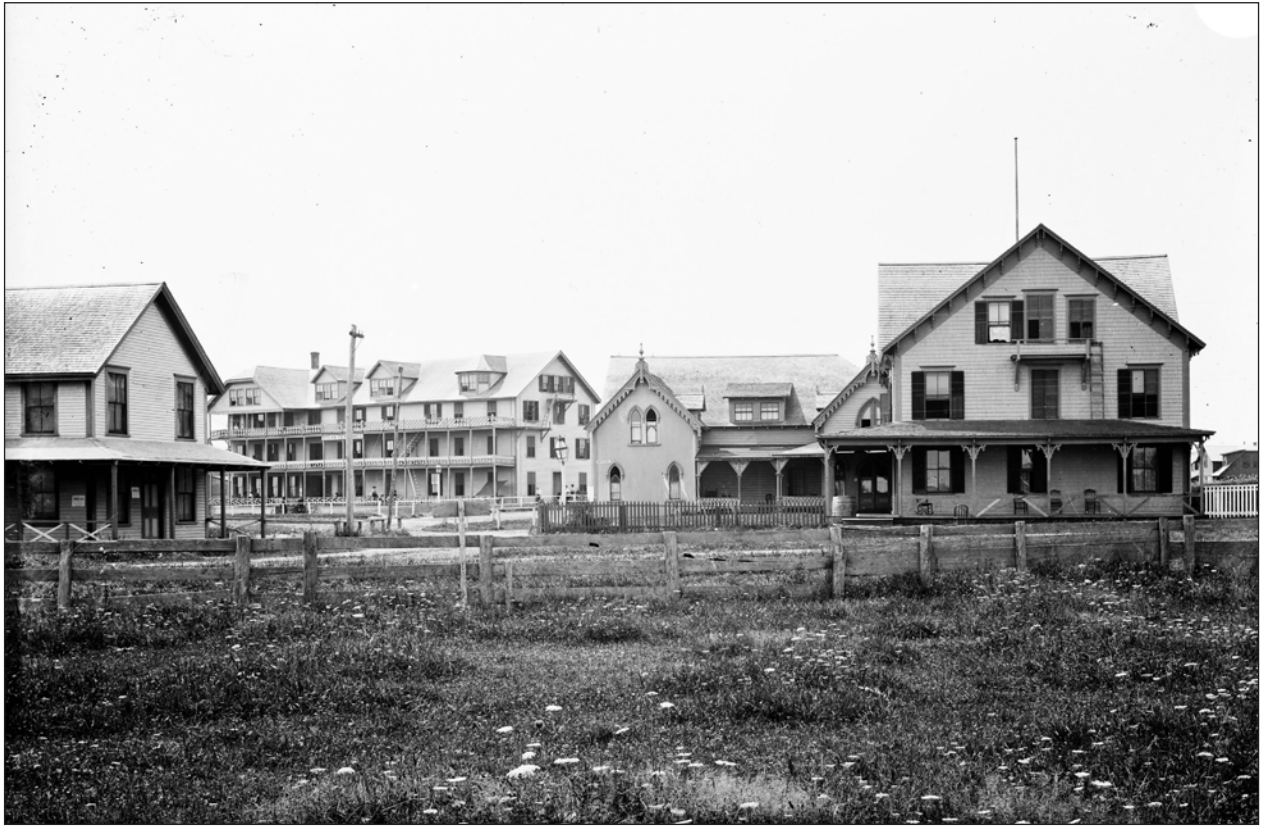
GPN 4149, Ocean View House and Annex, 1890s
