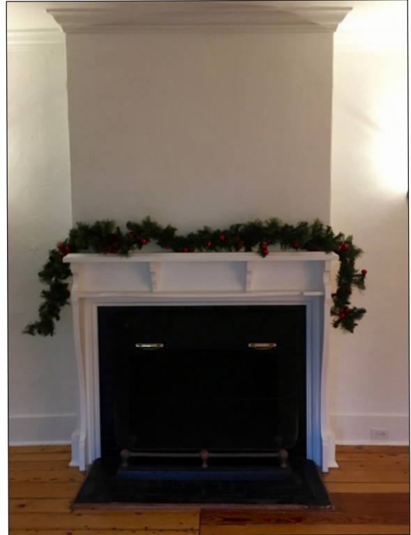
Fireplace, Northwest Room, 2020
