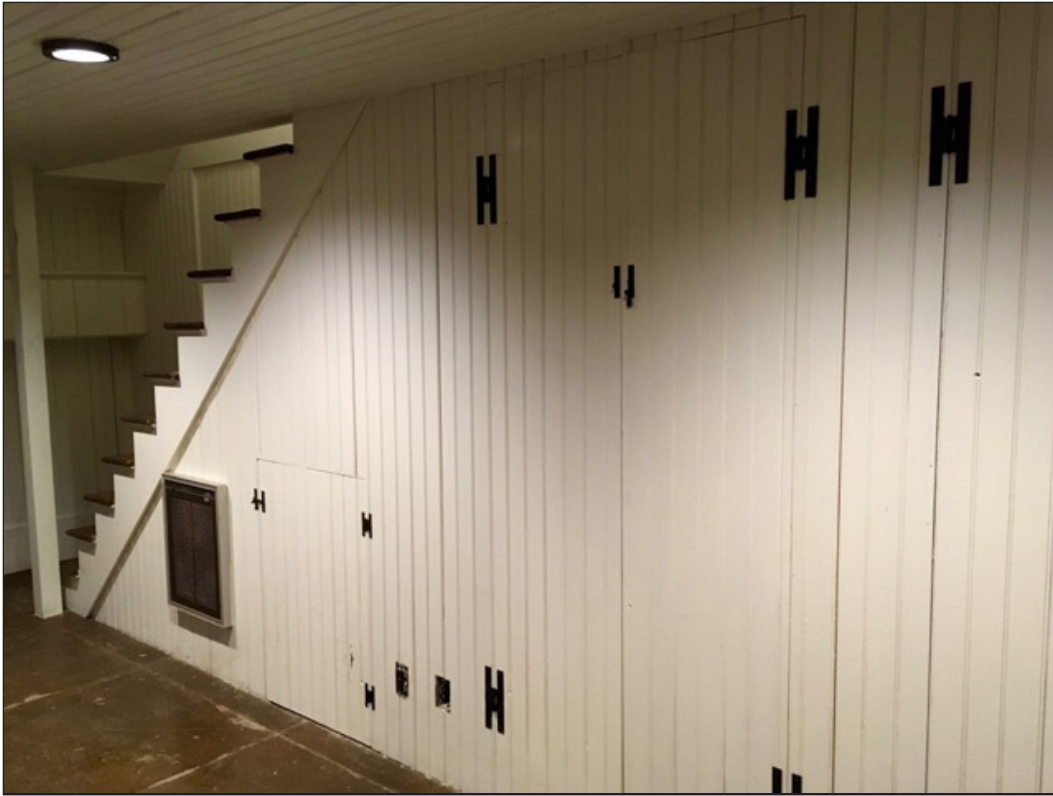
Wine Room in Partial Basement, 2020
