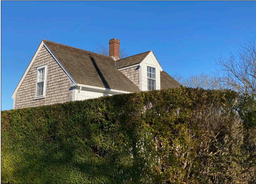
West Gable Elevation and South Dormer
