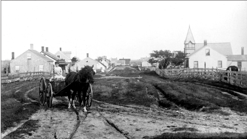
A15-11: Looking east, New Street is the third house on the left
