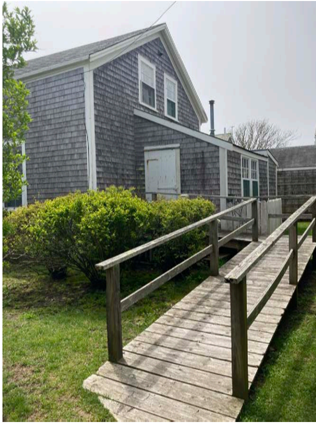
Ramp at Back North Door
