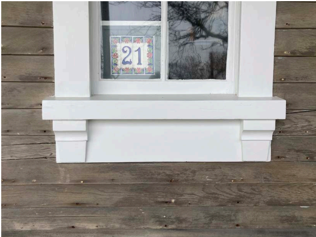
Original Round Arched Front Window Sill Detail
