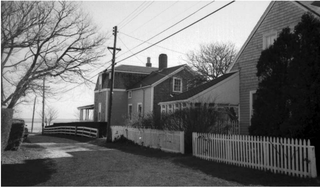
SC797-10: Magnolia Avenue looking east, 1960s: North and West Elevations
