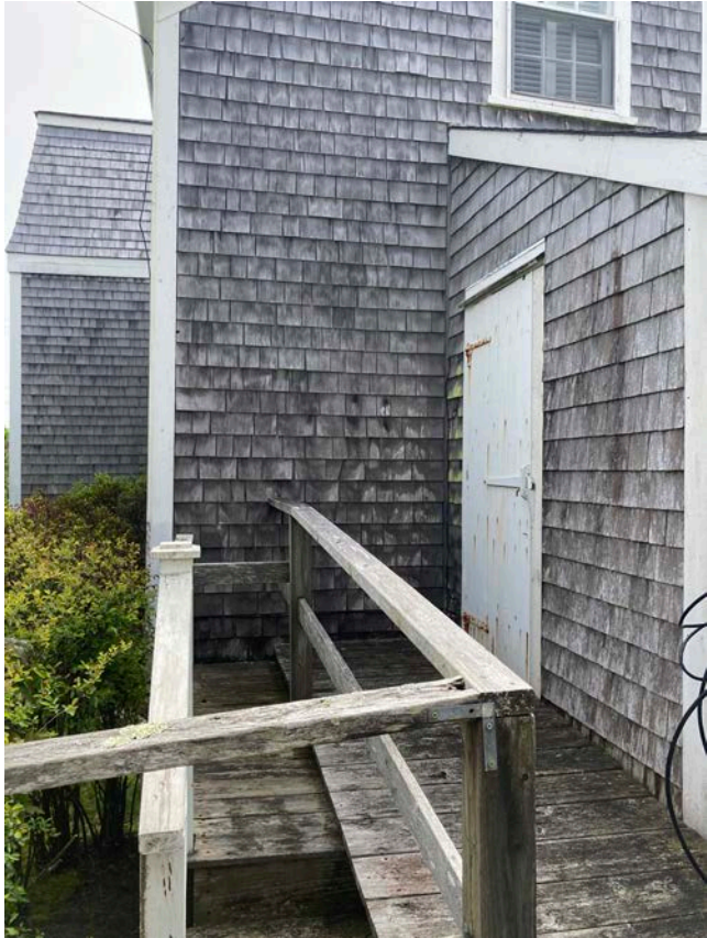
Ramp at Back North Door
