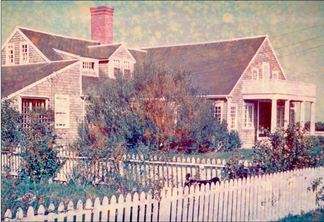
Heller O'Reilly Collection: Southwest elevations with rear gable and shed-roofed portions of original house
