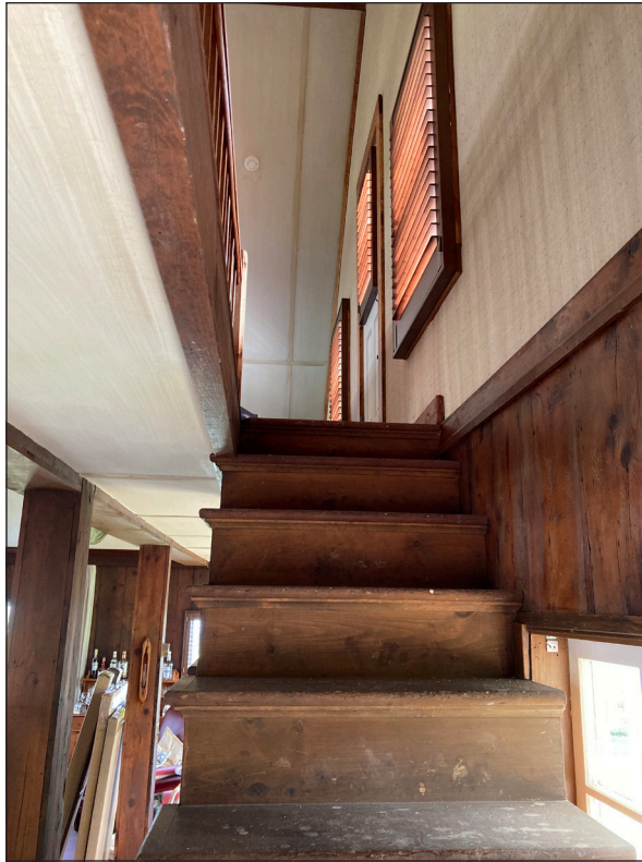
Stairs to Balcony, Performance Space
