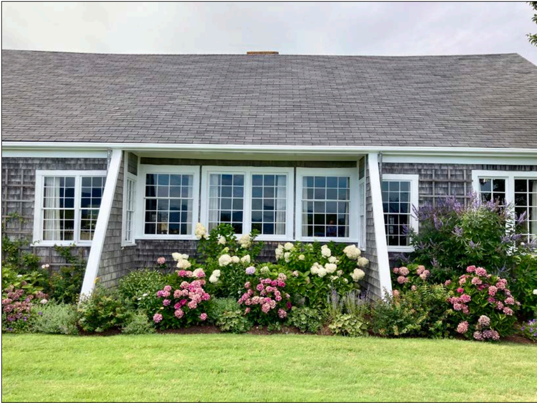
Buttress-like Walls, East Elevation
