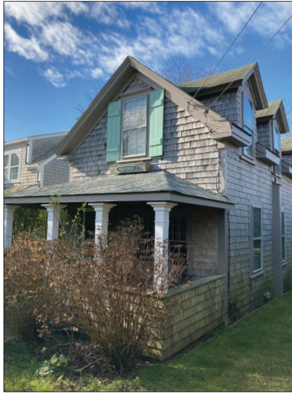
East/Front & North Elevations
