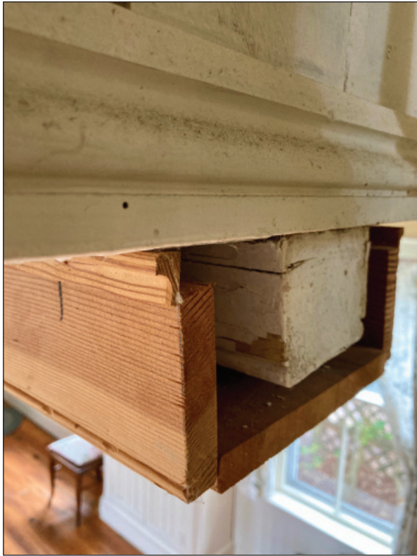
Living Room Ceiling Beam Cut
