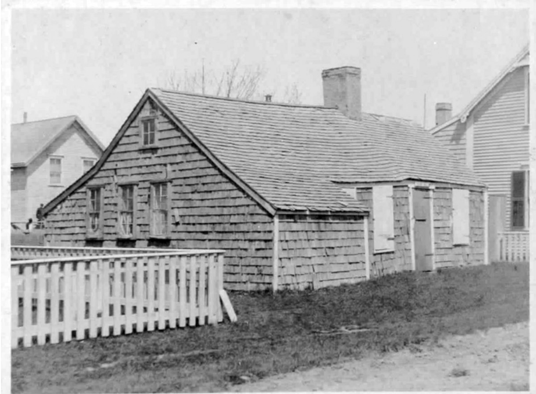
P2621: Auld Lang Syne, south façade, 1910s-20s Note the four plank-frame windows on the south elevation.
