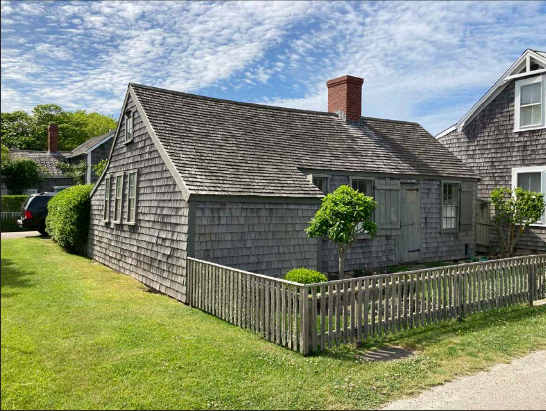
East/Front Broadway and South Elevations
