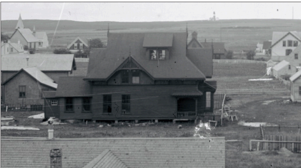
Close-up view of GPN526
