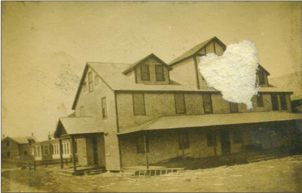
p20940: partial distant view of south elevation first floor windows, after 1909-1923
