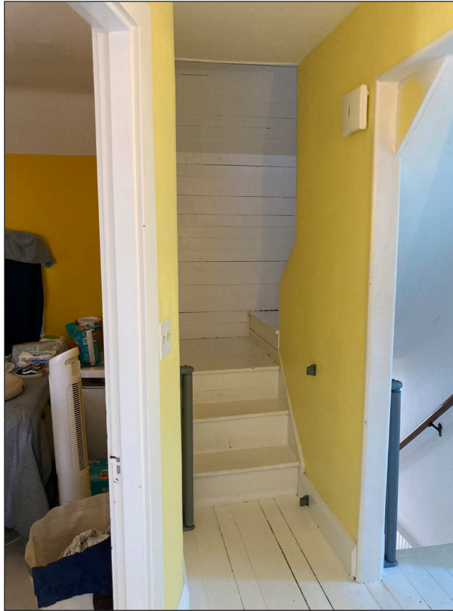
Second Floor Stair to Attic
