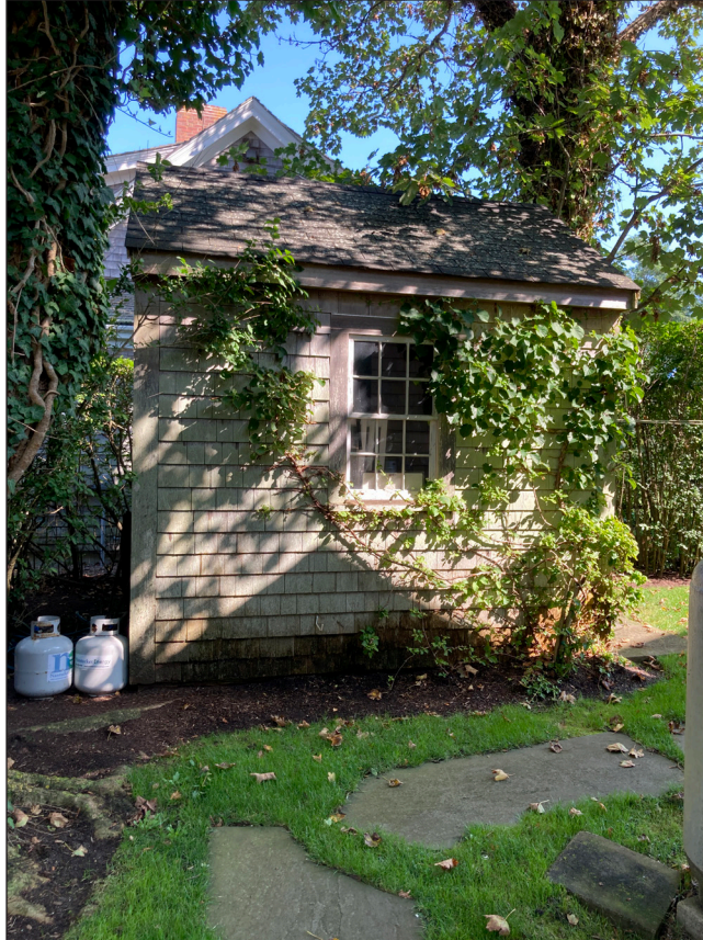
Shed at Northwest
