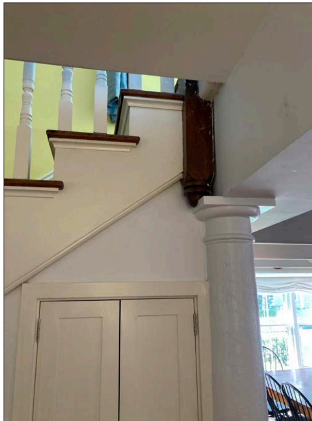
Front Hall Stair & circa 2000 Column
