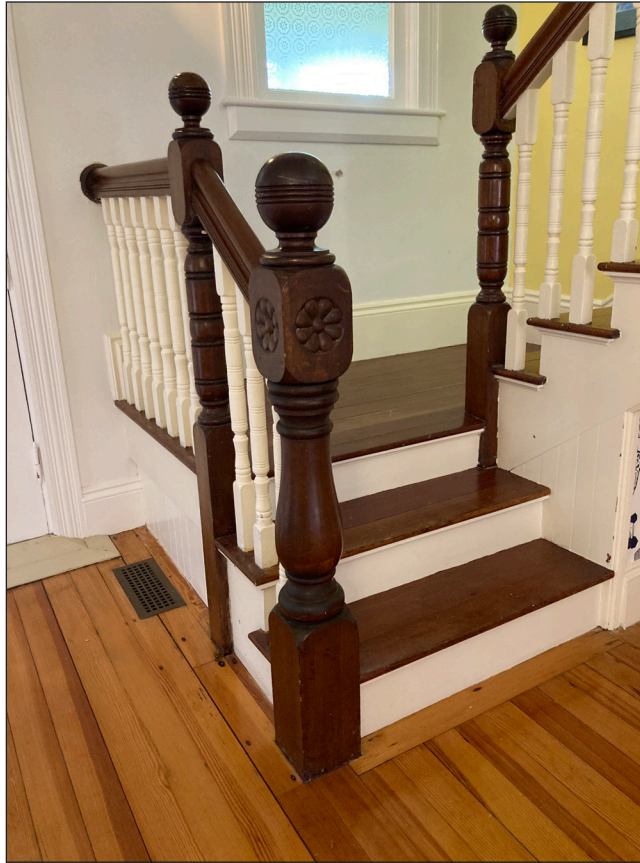
Front Hall Stair
